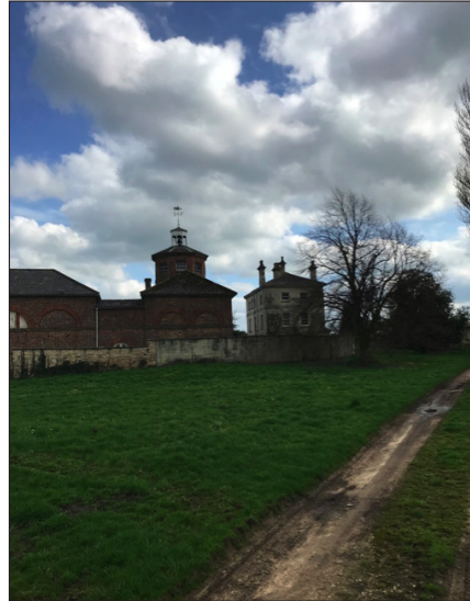
Outbuildings at Kirby Hall
