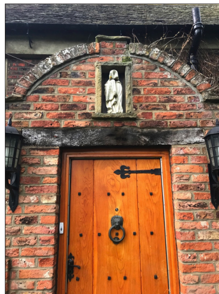
The monk above the front door
